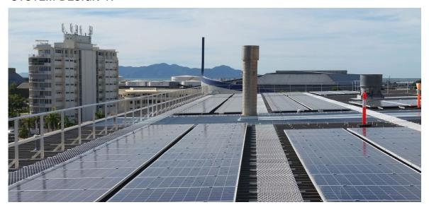
This installation shows walkway and handrail around the solar array. The walkway provides safe access to the individual panels while the Handrail protects from a fall edge.
